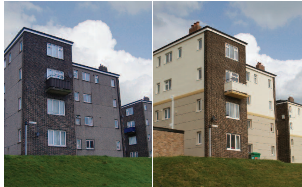
External improvements to Sowerby Road
